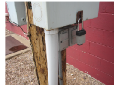
Detail showing existing GFI protected 110V outlet
